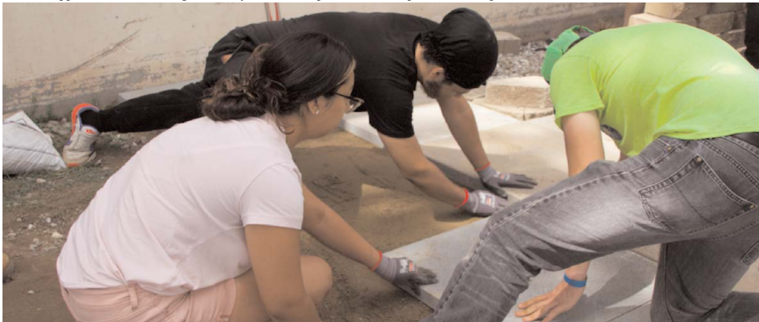
three student volunteers setting, leveling and caulking foundation paving stones that will hold the weight of stones above in finished sculpture garden.
