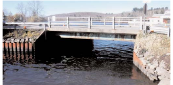
Sullivan County Bridge No. 51 spans the outlet of Swan Lake.
